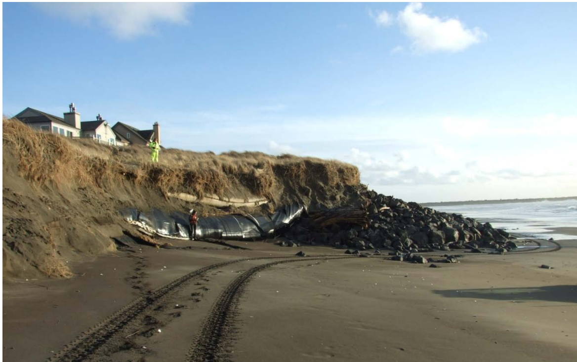
Figure 5. Dune erosion at Ocean Shores during winter 2010/2011 further exposed the rock revetment and geotubes that had been installed in 1996 and 1998 to protect condominiums and houses along this vulnerable shoreline reach.
